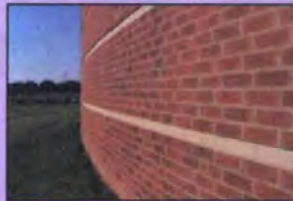
a brick wall / a wall made of bricks
